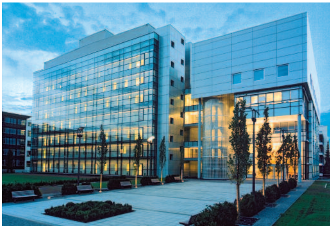
State of the art: manufacture of biopharmaceutical substances in Biberach. The “G 104” building is the largest single investment in the history of the company.
