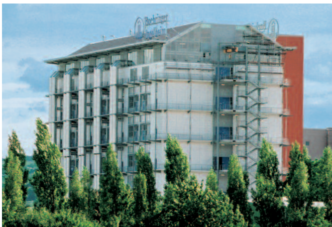
The 50 m high pharmaceutical active ingredients plant is designed as a multi-purpose plant for the synthesis of pharmaceutical substances. It was built in Ingelheim in 2003.
